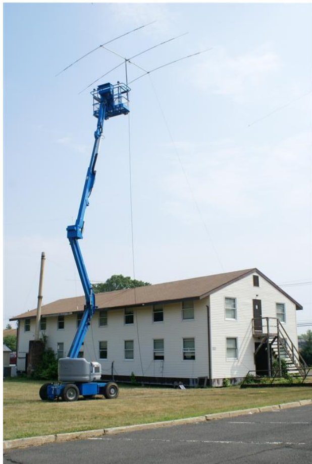
The Tri-band beam is up over 45 feet and worked out very well. It went up easily. The hardest part was bolting the elements to the boom. Picture by K2EI
